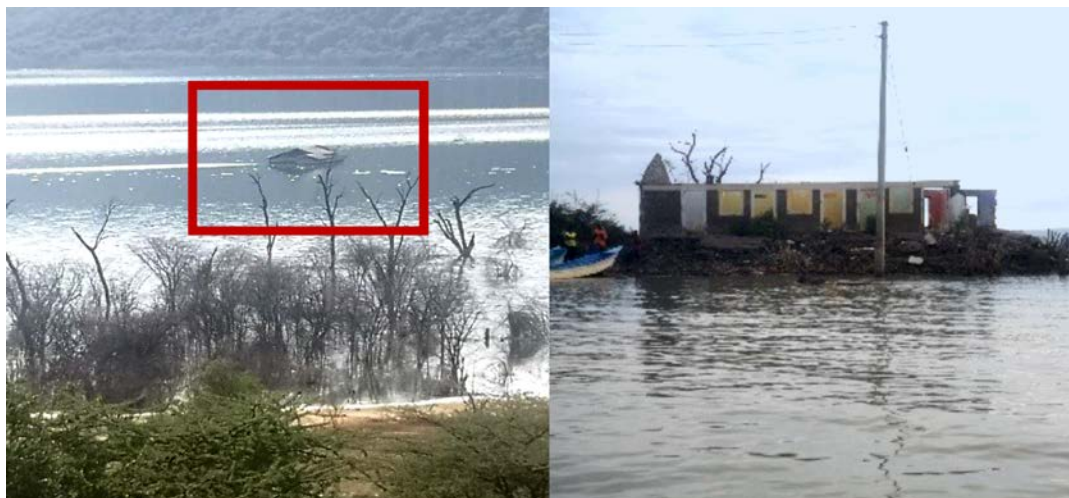
Figure 15: Houses destroyed by water in Lake Baringo.
